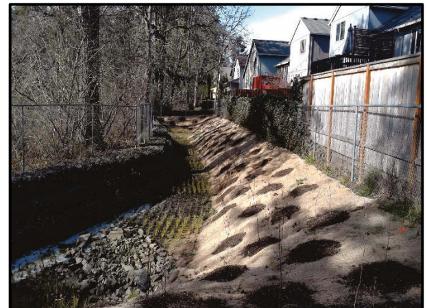
After: Facility was reshaped, planted, and rock was added. Photo was taken shortly after project completed.
