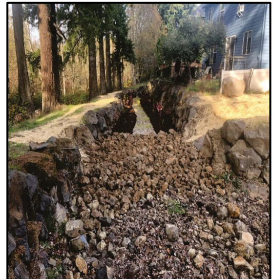
After: Depression is rocked and the swale is replanted.
