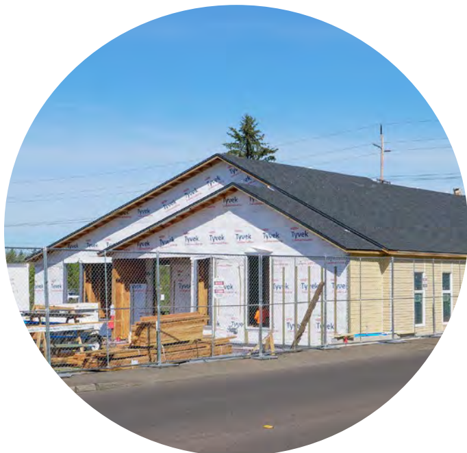
Year-Round Shelter Construction in Progress
