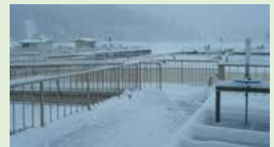
A snowy look at the Joint Water Commission Water Treatment Plant.
