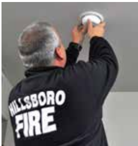
A Hillsboro firefighter installs a smoke alarm.
