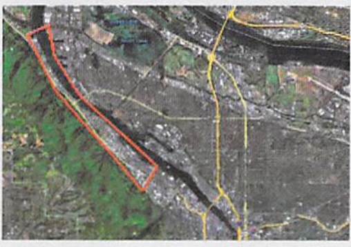
Left: Site map of the Critical Energy Infrastructure (CEI) Hub on the western bank of the Lower Willamette River area in NW Portland, Oregon. The CEI Hub, outlined in red, stretches for six miles. (Google Earth) Right: Oil terminals in the CEI Hub. (DOGAMI photo)
