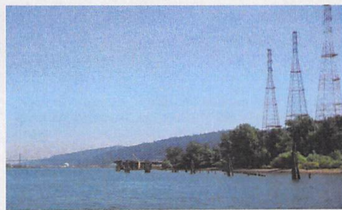
Left: These high voltage electrical transmission towers are built on a river bank in the Critical Energy Infrastructure (CEI) Hub susceptible to lateral spreading. (DOGAMI photo)
