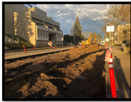
Remove underlying base rock.
