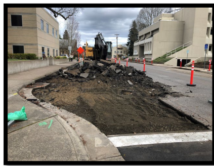
Remove existing paving.
