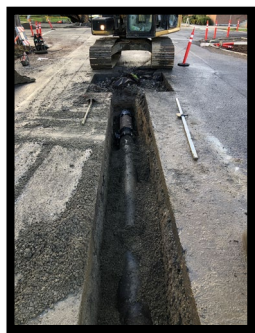
Install new utilities (if needed).
