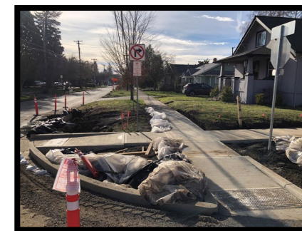
Build new curbs and ramps.
