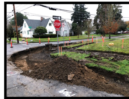
Remove curbs and curb ramps.
